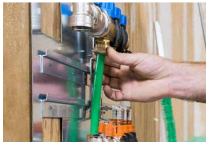
Connecting the underfloor heating pipes to the manifold, filling the system with water and leakage test.
