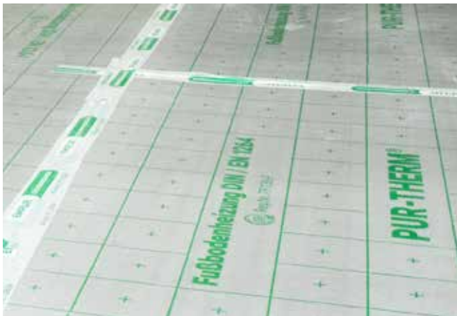
Laying of EMPUR® composite panels. The single-sided film overhang overlaps the connecting panel and prevents the penetration of screed.
