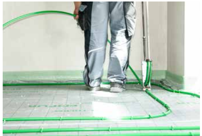
Installation of the KLIMAPEX® heating pipes using the preprinted laying grid with PUR-THERM® staples and the system tacker.
